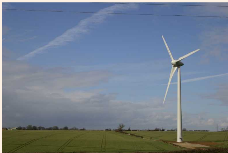
Wind Turbine at Burton Wold Wind Farm
