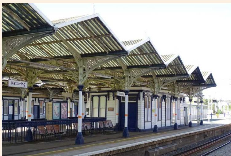
Kettering Train Station
